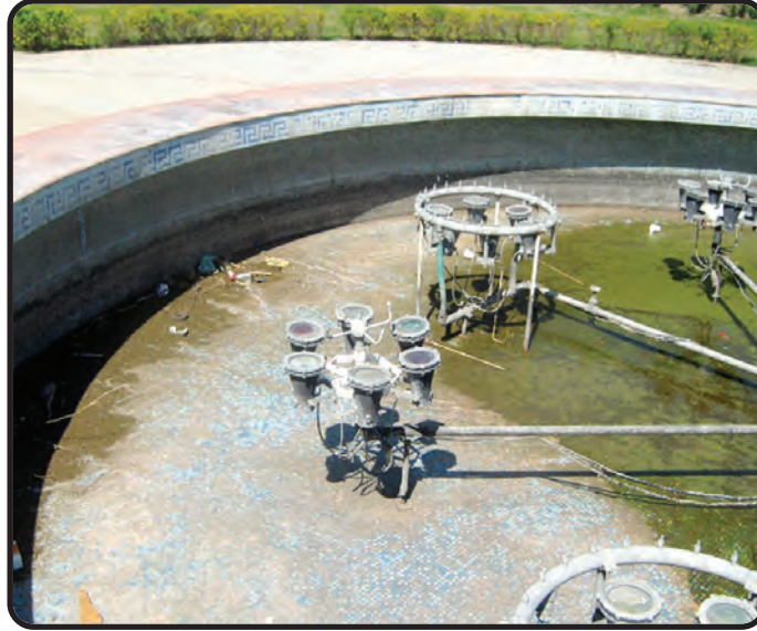
Dry Foundations at the Memorial
