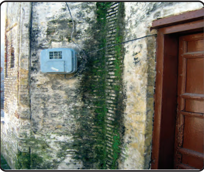
Electric wires hanging loose - an invitation to accident
